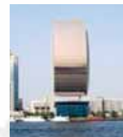
National Bank of Dubai, Dubai, U.A.E.
