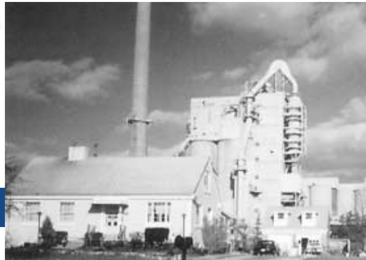
Figure 1: Example of industrial facility located near a residence
